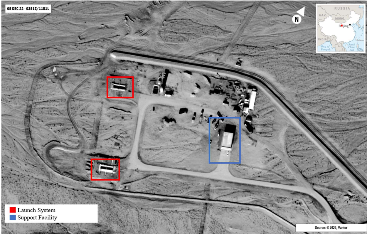
Image 2: Construction of launch site in December 2022, launchers do not have closure doors installed.
